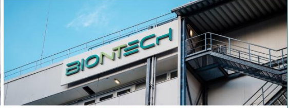
Bulk mRNA production facility, Marburg, Germany
