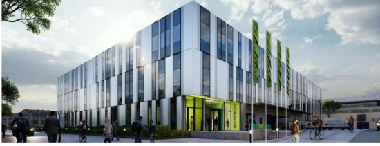
Personalized mRNA production facility, Mainz, Germany
